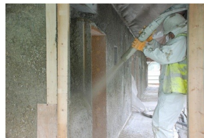
Figur 5 LHC sprayning (CAT,2013)
