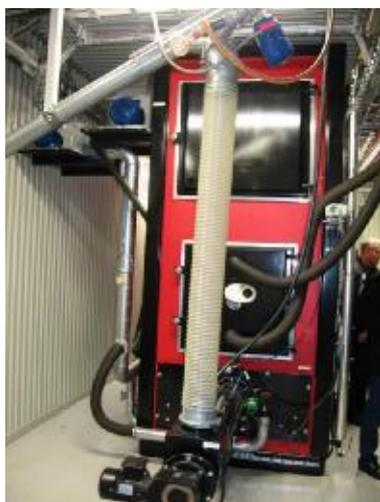
Figure 2. New main boiler of 1500kW fuelled with pellets (Stepfire by TPS).
