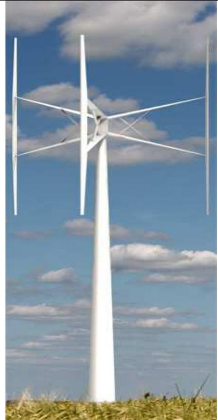
The tower is built of wood composites instead of steel or concrete. The composites consist of fiberglass and wooden beams. The material provides environmental and technical advantages.
