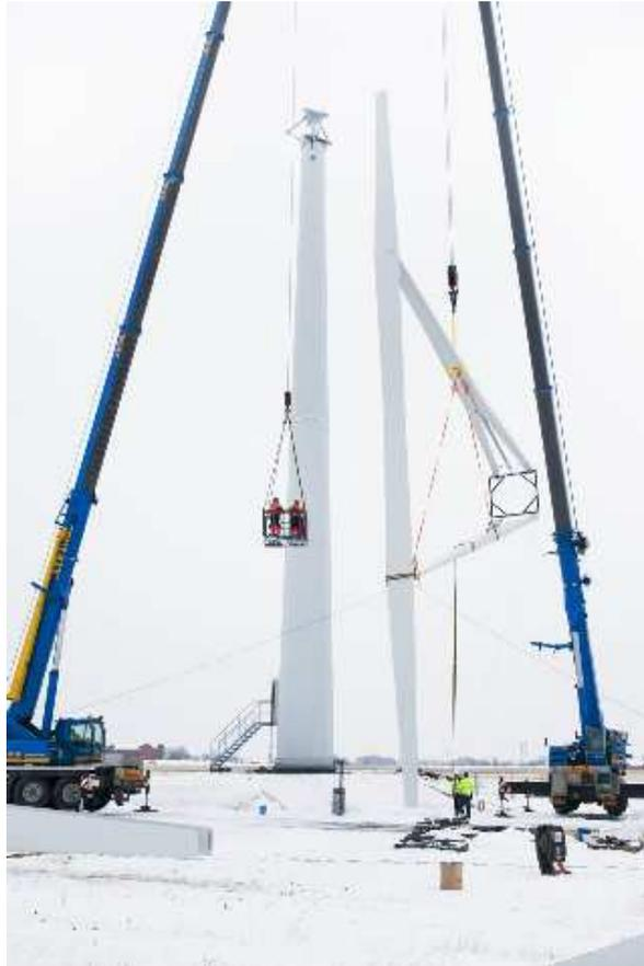
*In the winter 2010 the first 200 kW vertical axis wind turbine manufactured by Vertical Wind AB was erected in Falkenberg. Photo: Lars Owesson*
